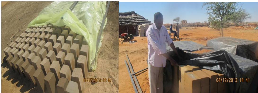
Stabilized soil blocks (SSB) production for construction of the classrooms
