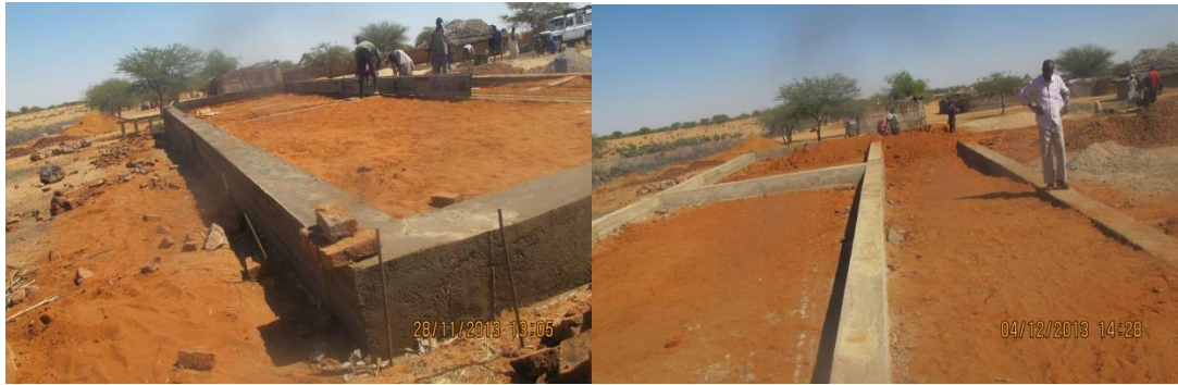
2 classrooms construction(foundation work) , Umkadoia West School for Girls in Umdam village
